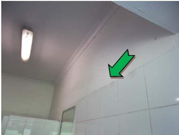
Photo 3. Interior, unisex toilet, walls – non asbestos-containing fibre cement sheeting.
