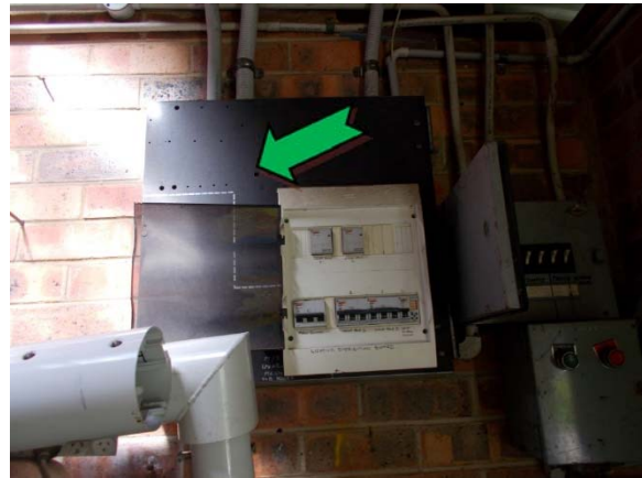
Photo 4. Interior, store room, switchboard - non asbestos-containing bituminous backing board.
